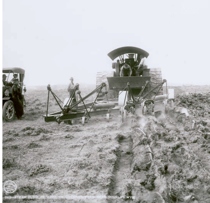
Steam plow on Unland's farm, Douglas. This steam tractor is the same device that would power threshing machines; here it is breaking sod. The huge machine required two operators on board, both visible in this photograph. Photo: J. E. Stimson Collection, Wyoming State Archives, negative 2925.
