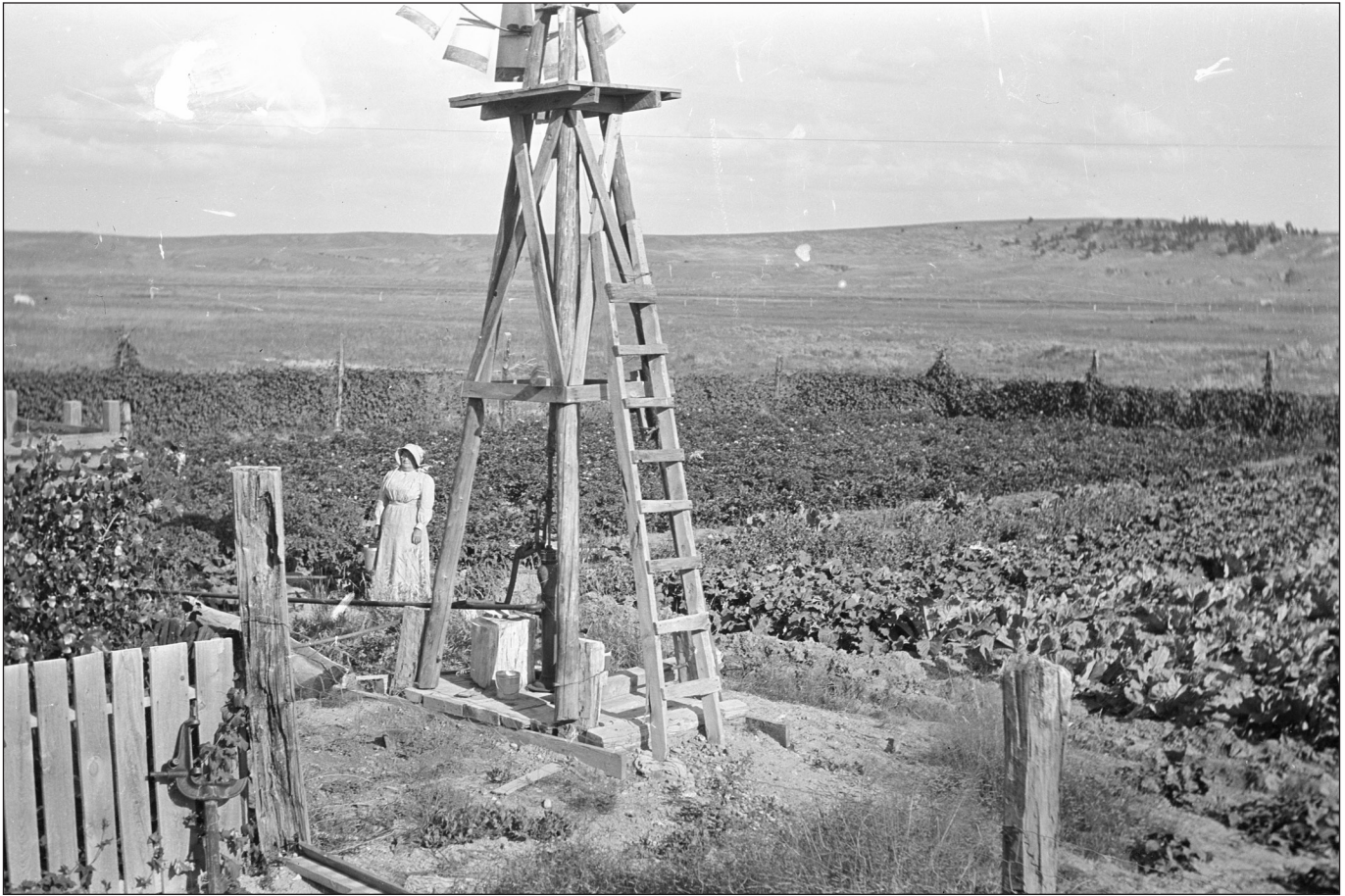
Although windmills are often associated with open prairies and ranges, they were also an integral part of many ranch and farmsteads. This undated image from the Roy Hook Ranch in Uinta County shows the operating mechanism of the windmill below the platform, including the pump (and pipe for diverting water for domestic use, irrigation, or storage), and a wooden tower. The presence of the integral ladder indicates that the windmill possibly predated the self-oiling systems. Photo: Roy Hook Ranch Photographs and Negatives, 1902-1913, American Heritage Center, University of Wyoming.
