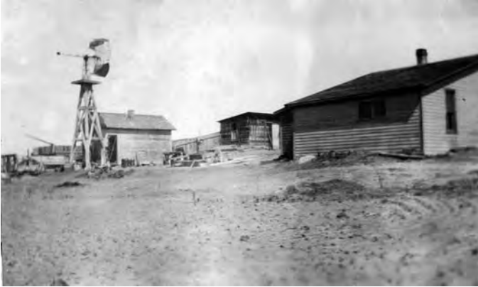
Tadewald house made from 3 homestead shacks, 1926
