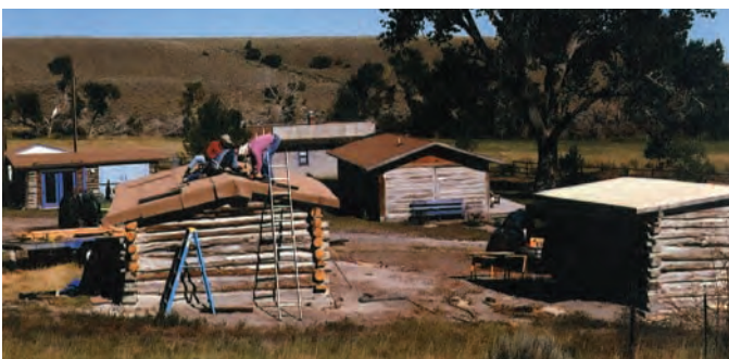
Quien Sabe Ranch, re-roofing bunk house
