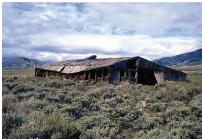
Shearing Shed built in 1920 by John Cheesbrough, still standins
