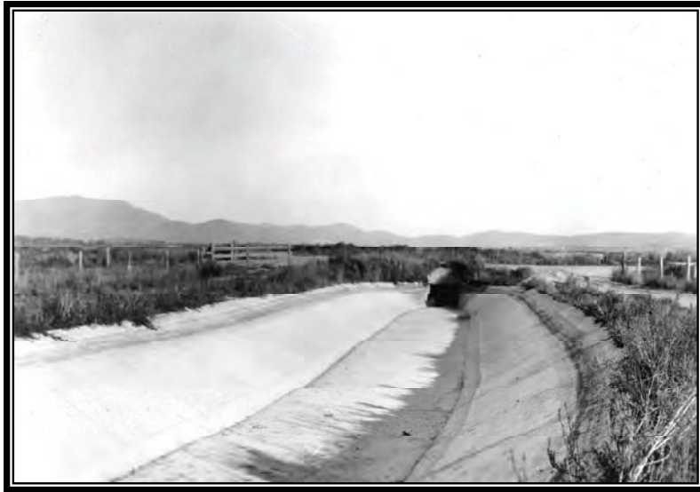
Camp BR-20: Klamath Project, concrete lining constructed by CCC enrollees at head of J-1 Lateral, 1937 (Box 61, Entry 10, RG 115, National Archives, Denver).
