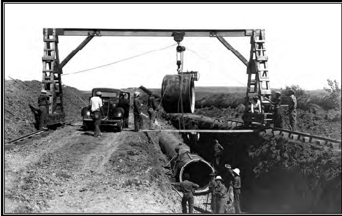
Camp BR-2: Belle Fourche Project, installing North Canal Siphon, June 23, 1936 (Box 23, Entry 10, RG 115, National Archives, Denver).
