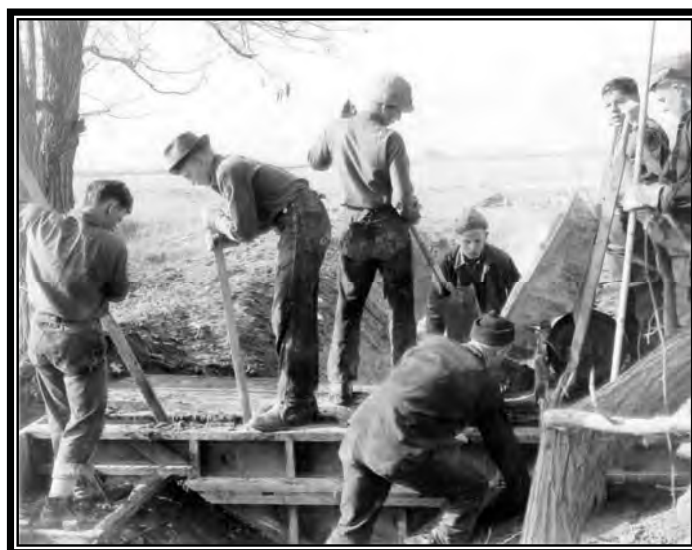
Camp BR-24: Boise Project, enrollees placing a lateral drop, February 8, 1940 (Box 1, Entry 31, RG 115, National Archives, Denver).
