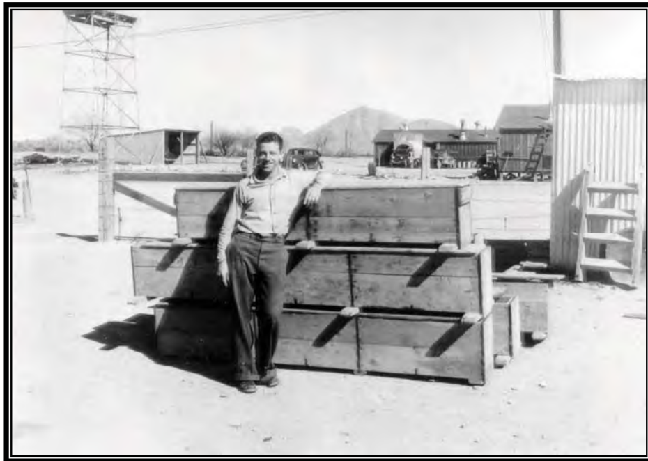
Camp BR-14: Salt River Project, removable tool boxes that are also used for seats in trucks, March 23, 1937 (Box 15, Accession No. 8NS-115-95-112, RG 115, National Archives, Denver).
