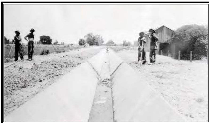
Camp BR-13: Yuma Project, concrete precast slabs placed in Woods Lateral, September 20, 1939 (Box 1, Entry 31, RG 115, National Archives, Denver).
