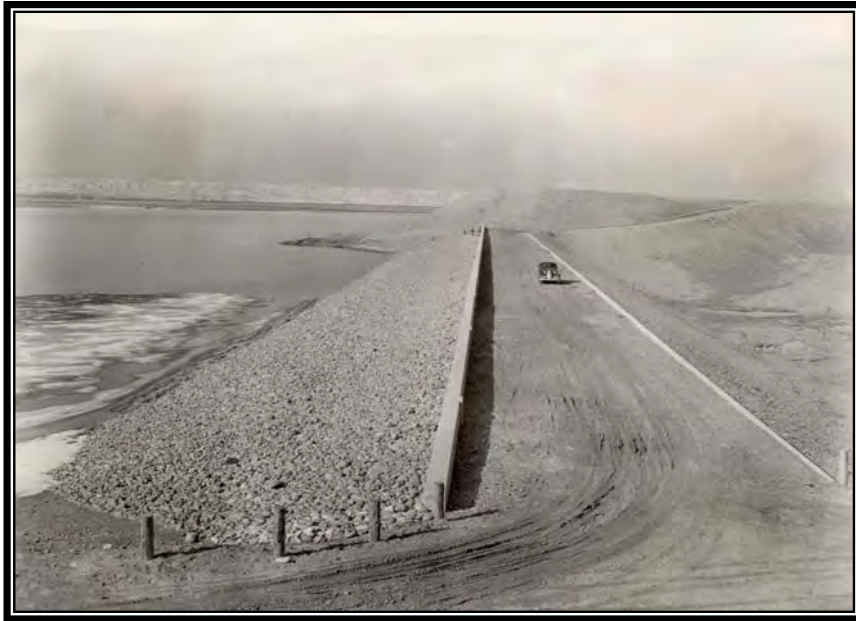
Camp BR-11: Moon Lake Project, completed parapet and curb walls on Midview Dam, March 29, 1940 (Accession No. 8NN-115-90-011, RG 115, National Archives, Denver).
