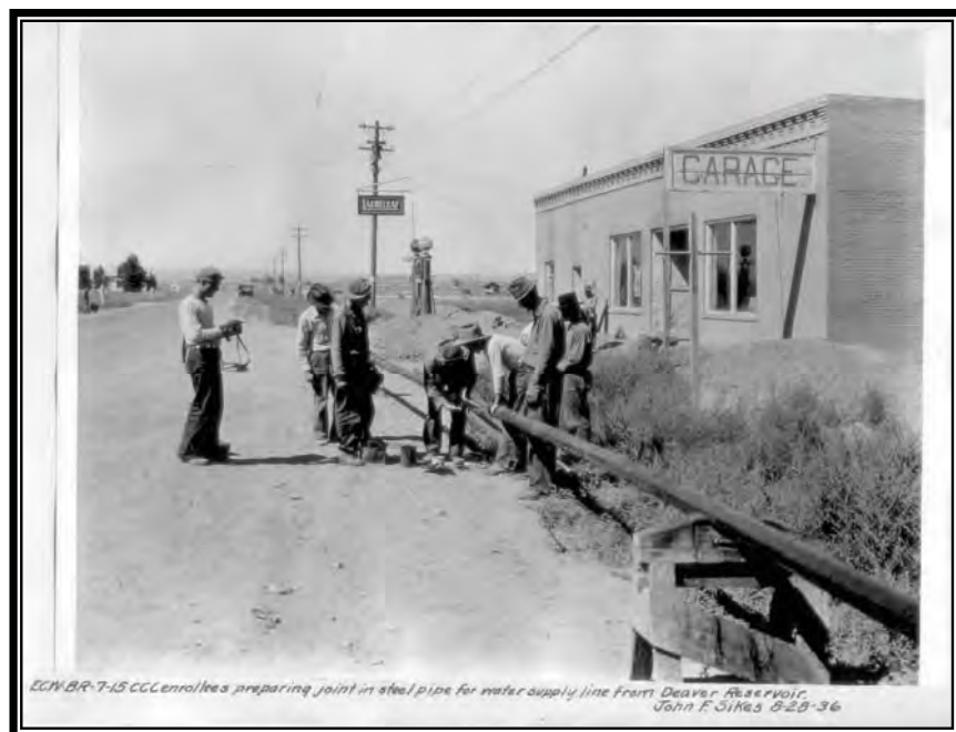
Camp BR-7: Shoshone Project, enrollees preparing joint in steel pipe for water supply from Deaver Reservoir, August 28, 1936 (courtesy of Shoshone Irrigation District).
