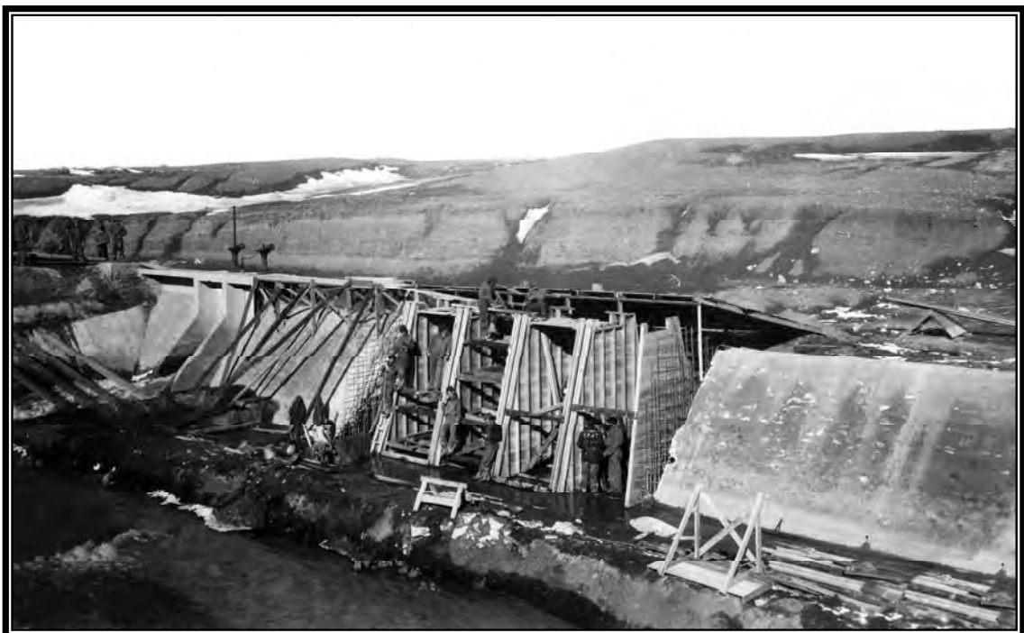
Camp BR-2: Belle Fourche Project, form work for check reservoir drop, November 19, 1936 (Box 23, Entry 10, RG 115, National Archives, Denver).
