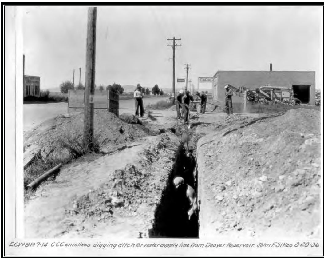
Camp BR-7: Shoshone Project, enrollees digging ditch for water supply line from Deaver Reservoir, August 28, 1936 (courtesy of Shoshone Irrigation District).
