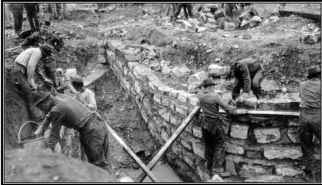
Camp BR-23 and BR-71: Uncompahgre Project, placing rock and mortar in check in Spring Creek, April 21, 1941 (Box 1, Entry 31, RG 115, National Archives, Denver).
