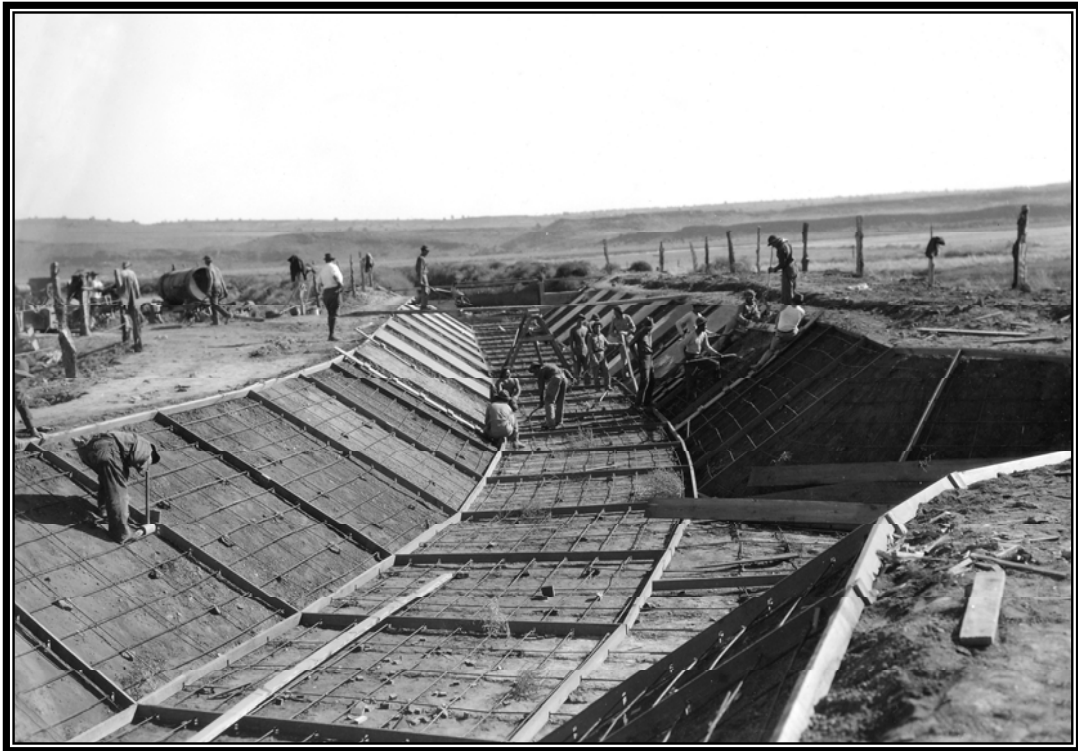
Camp BR-20: Klamath Project, CCC enrollees lining J Canal near Bloody Point, 1937 (Box 161, Entry 10, RG 115, National Archives, Denver).
