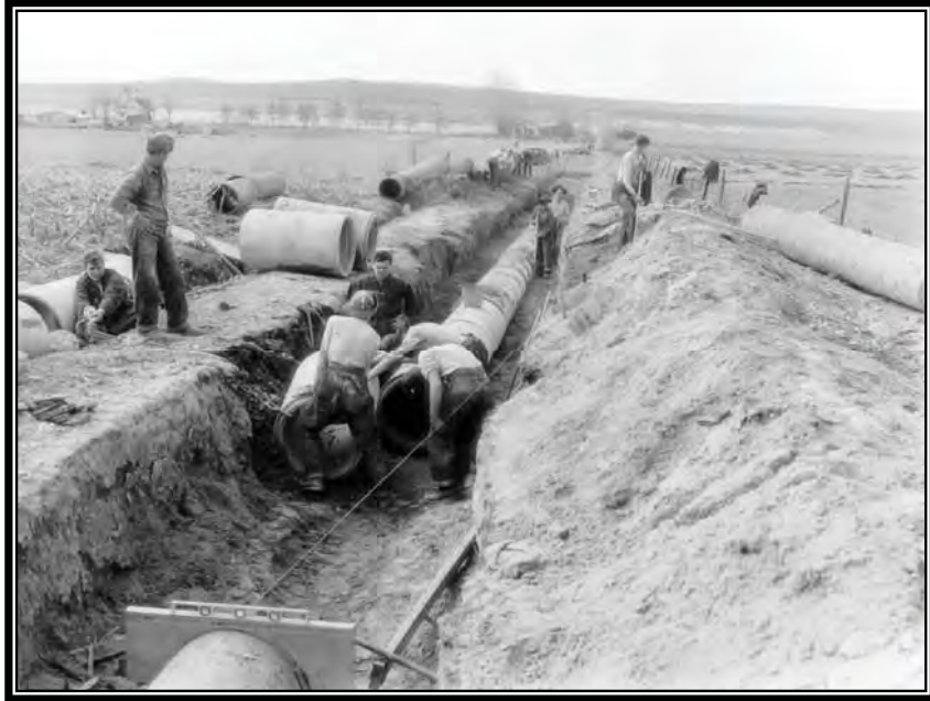
Camp BR-24: Boise Project, crew placing 24-inch concrete pipe, March 14, 1941 (Box 1, Entry 31, RG 115, National Archives, Denver).
