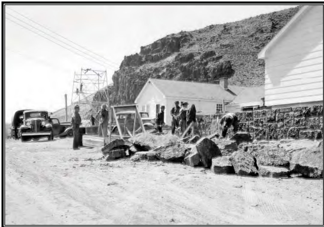
Camp BR-20: Klamath Project, rock wall construction at wildlife refuge headquarters, date unknown (Box 1, Entry 31, RG 115, National Archives, Denver).
