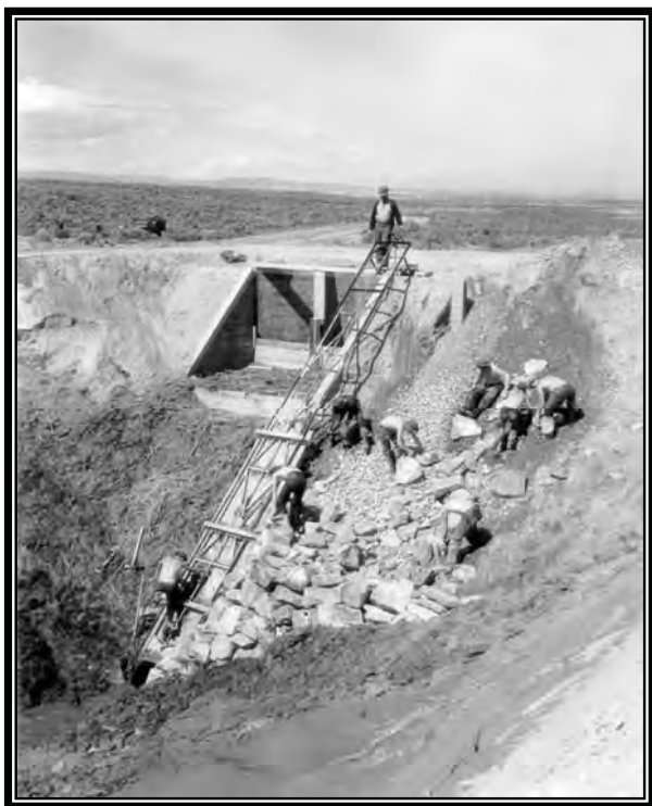
Camp BR-24: Boise Project, enrollees placing gravel and rock riprap around inlet of overflow pipe in Gem Irrigation District drain, April 3, 1940 (Box 1, Entry 31, RG 115, National Archives, Denver).
