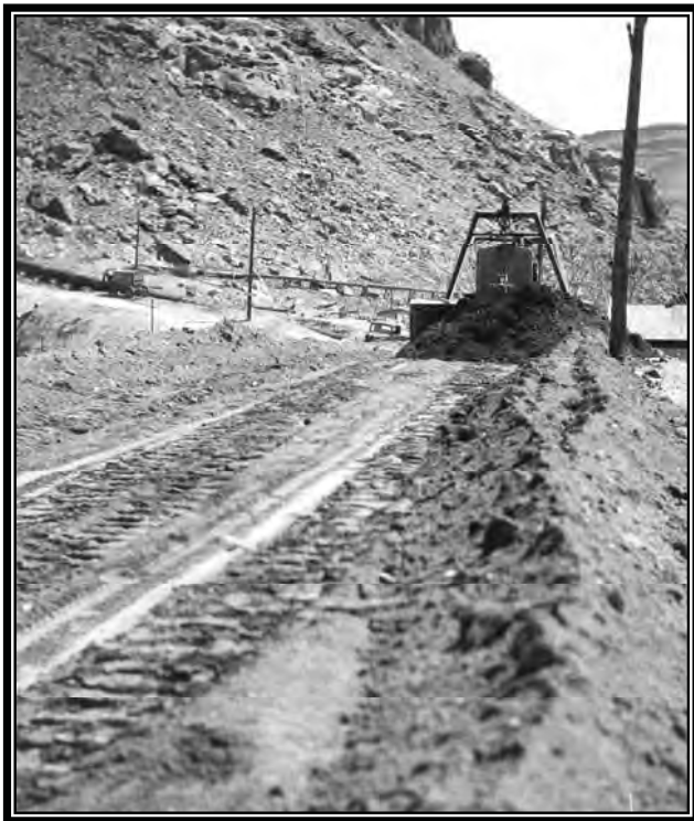
Camp BR-22: Grand Valley Project, angledozer widening canal banks near Palisade for road purposes, 1938 (Box 320, Accession No. 8NN-115-90-011, RG 115, National Archives, Denver).
