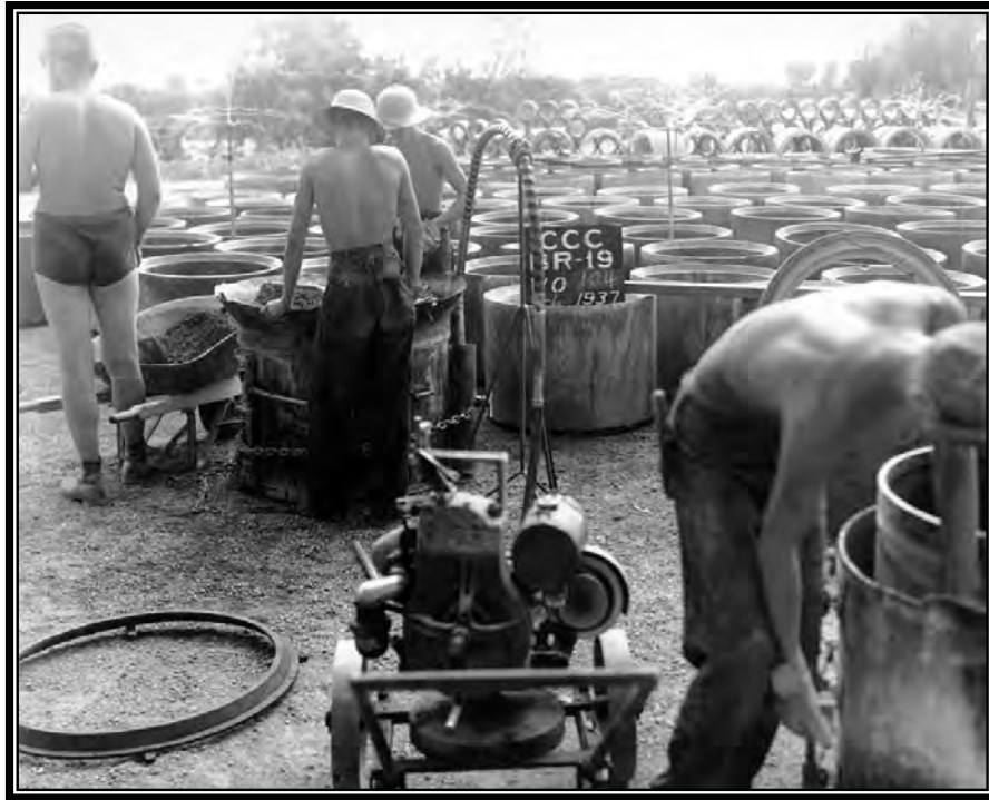
Camp BR-19: Salt River Project, manufacturing concrete pipe, 1937 (Box 143, Entry 22, RG 115, National Archives, Denver).
