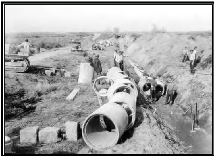
Camp BR-24: Boise Project, enrollees placing concrete pipe siphon on lateral system, 1939, (Box 39, Entry 10, RG 115, National Archives, Denver).
