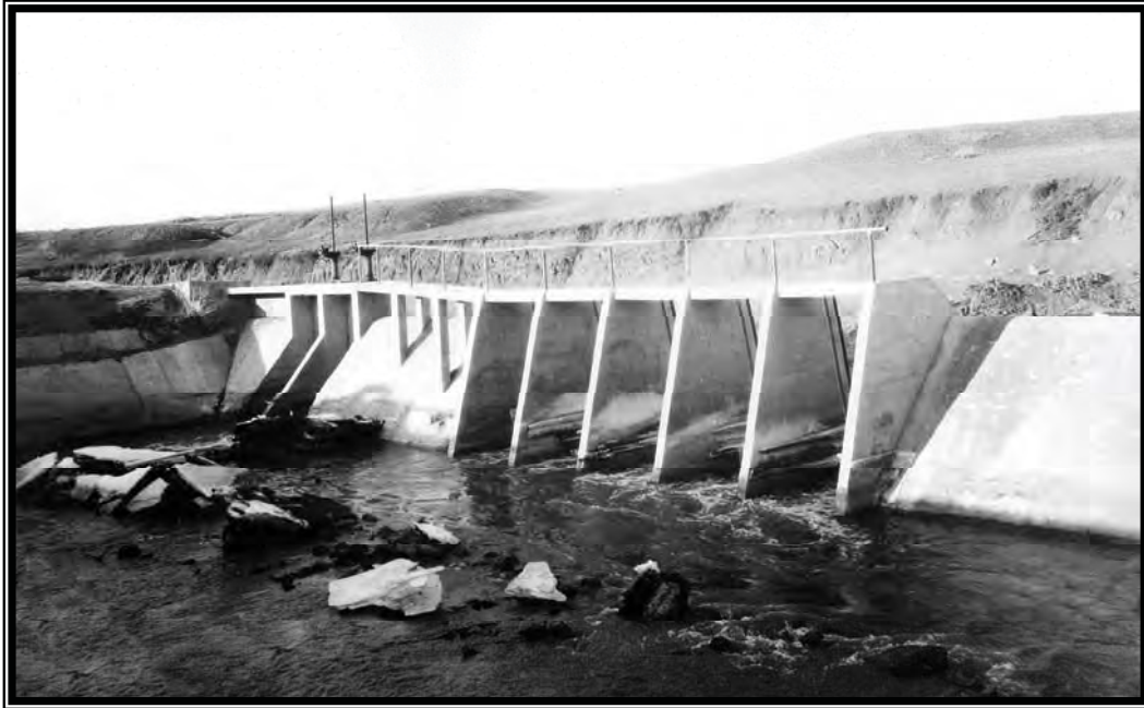
Camp BR-2: Belle Fourche Project, new check outlet-reservoir drop, December 15, 1936 (Box 23, Entry 10, RG 115, National Archives, Denver).
