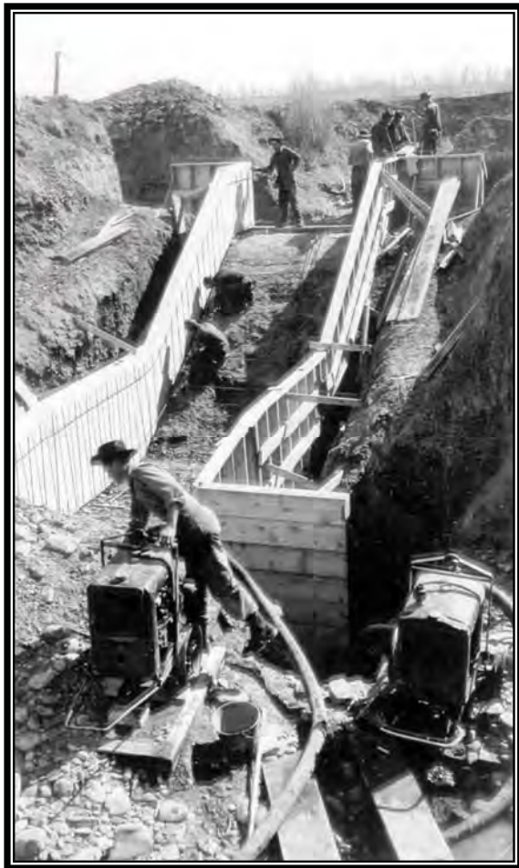
Camp BR-23 and BR-71: Uncompahgre Project, setting forms for the F.L.-3.25 concrete check, March 18, 1941 (Box 1, Entry 31, RG 115, National Archives, Denver).
