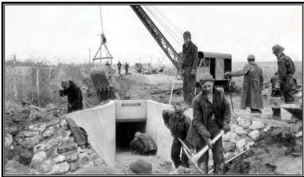
Camp BR-23 and BR-71: Uncompahgre Project, backfilling around completed concrete pipe siphon at C.Q.A.-0.86, February 9, 1940 (Box 1, Entry 31, RG 115, National Archives, Denver).
