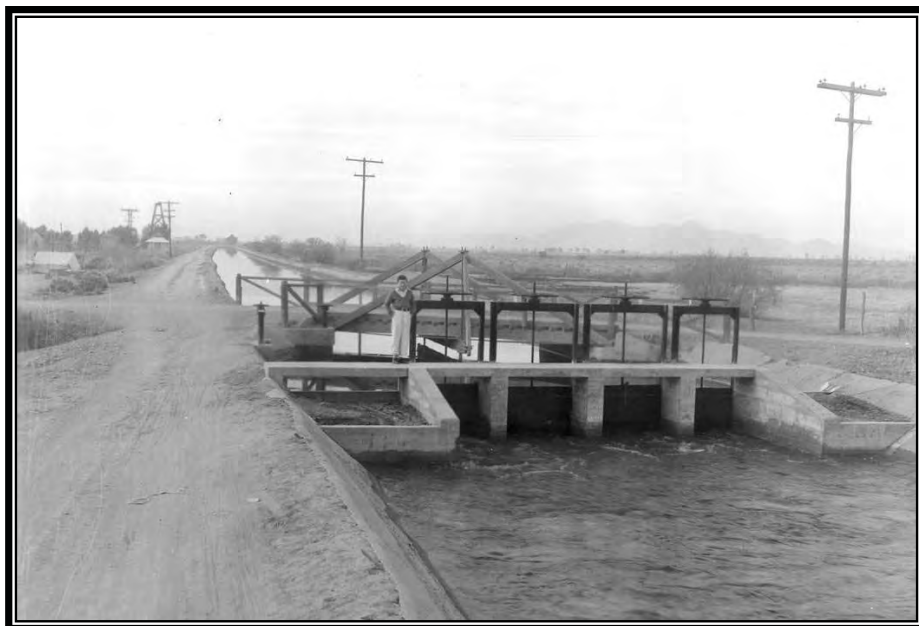
Camp BR-14 and BR-19: Salt River Project, new Eastern Canal gate structure, date unknown (Box 143, Entry 22, RG 115, National Archives, Denver).
