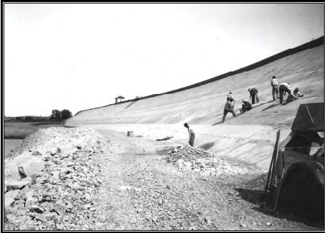
Camp BR-2: Belle Fourche Project, repairing revetment, Belle Fourche Dam, 1940 (Box 23, Entry 10, RG 115, National Archives, Denver).
