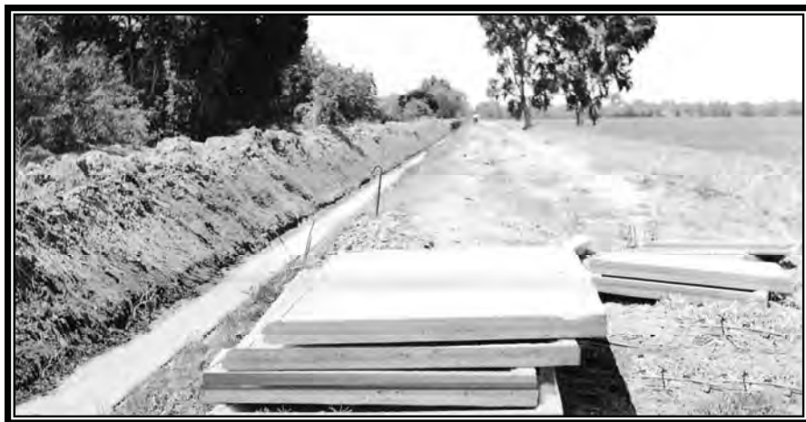
Camp BR-13: Yuma Project, placing precast concrete slabs in Woods Lateral, September 20, 1939 (Box 1, Entry 31, RG 115, National Archives, Denver).
