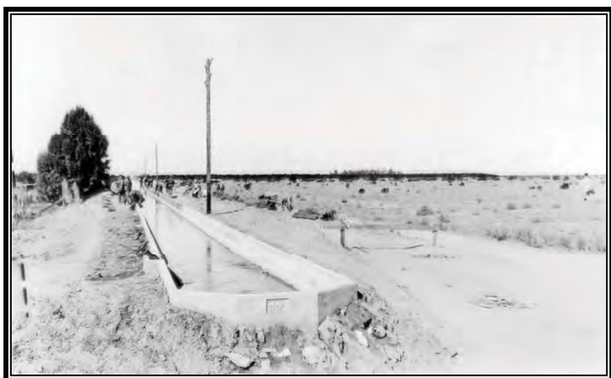
Camp BR-13: Yuma Project, raising concrete lining, B-8 Lateral, Yuma Mesa, March 15, 1940 (Box 1, Entry 31, RG 115, National Archives, Denver).
