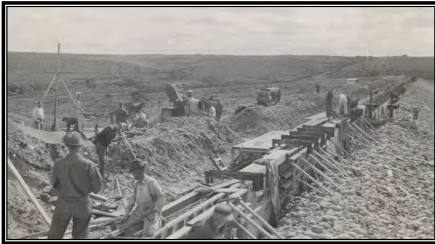
Camp BR-11: Moon Lake Project, concreting operations for parapet wall at Midview Dam (Box 97, Accession No. 8NN-115-90-011, RG 115, National Archives, Denver).
