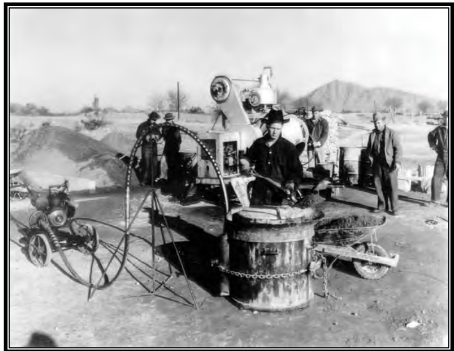
Camp BR-19: Salt River Project, gasoline driven concrete vibrator, January 26, 1937 (Box 15, Accession No. 8NS-115-95-112, RG 115, National Archives, Denver).
