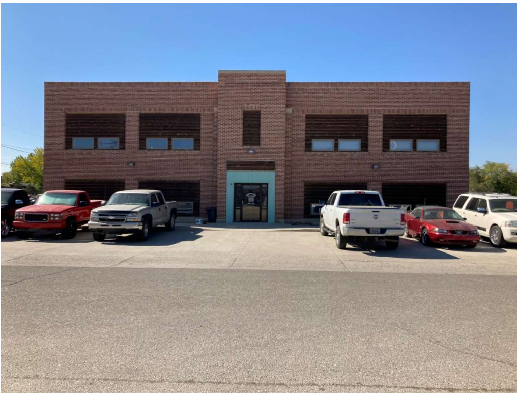
Figure 7 Front view of former Mexican/Spanish School, 2021
