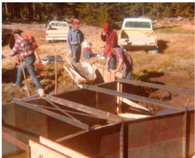
Community members working on Parshall flume below the new Shoshone Lake dam. 1958.
