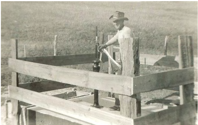
Keith installing a new water pump over the hand dug well.
