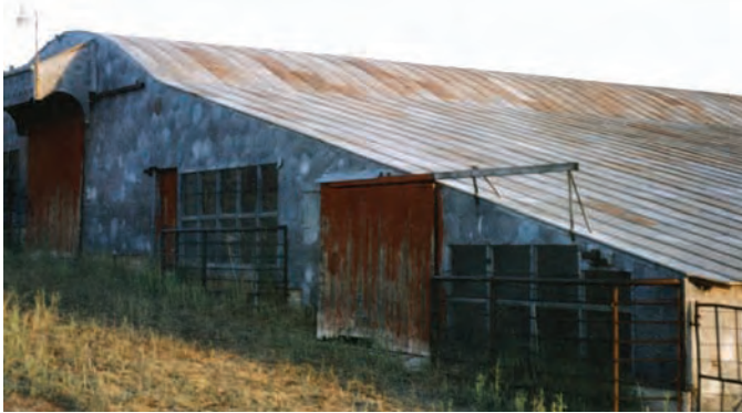
Former lambing shed, now a calving shed. Roof is recycled sides of cans, processed with the machine Carl designed & built specifically for this purpose.
