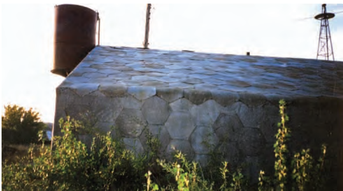
Old shop still filled with Carl's machinery & equipment inventions; sided and roofed with can bottoms
