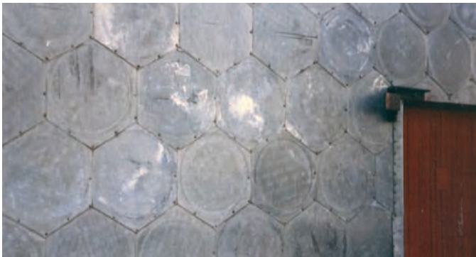
Buildings on ranch sided & roofed with recycled cyanide cans purchased from Homestake Gold Mine in Lead, SD
