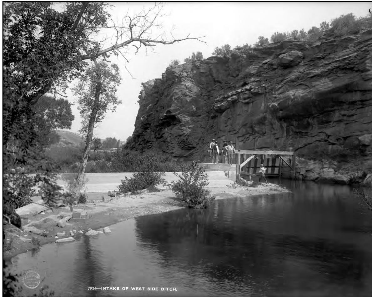
Figure 7. Example of the intake structure, circa 1909, of the West Side Ditch by the North Platte Valley Irrigation Company. Intake West Side Ditch, J.E. Stimson Collection, STIMSON NEG 2934, Wyoming State Archives.
