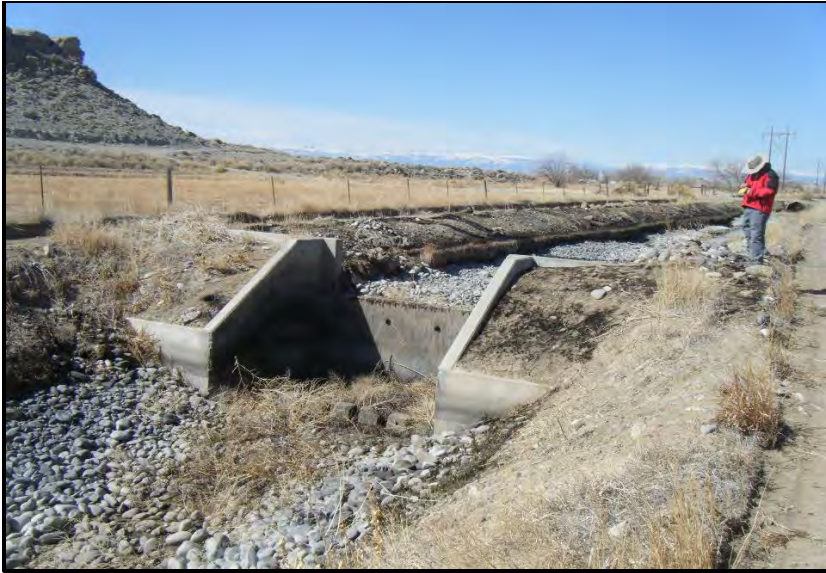
Figure 67. Example of a protective weir on the Fivemile Lateral in Fremont County.
