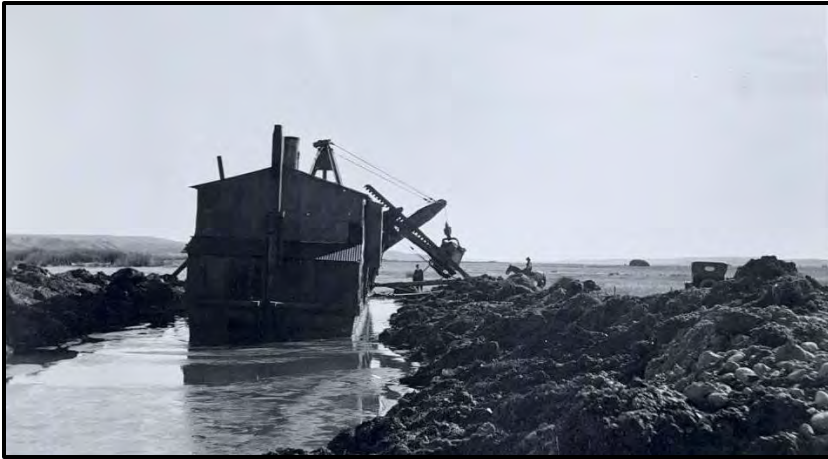
Figure 44. Historical photograph, unknown date, of a steam-powered shovel cleaning out, or dredging, the Green River Canal. Green River Canal, Irrigation #2 of 3, IRRIG 31, Wyoming State Archives.
