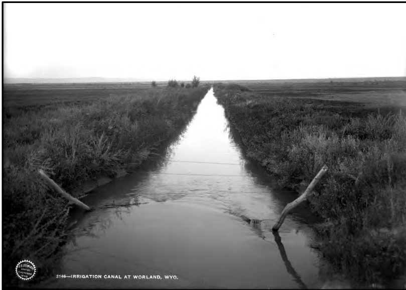
Figure 5. An undated historical photograph of an open, earthen ditch used to convey water through pasture and fields near Worland, Wyoming. Irrigation Canal, Worland WY, J.E. Stimson Collection, STIMSON NEG 3146, Wyoming State Archives.
