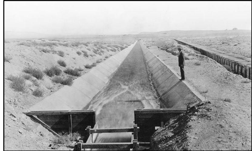
Figure 43. Portion of a concrete-lined canal associated with the Shoshone Project, unknown date. Canal carrying water, Kuska Collection, P72-79/1019, Wyoming State Archives.
