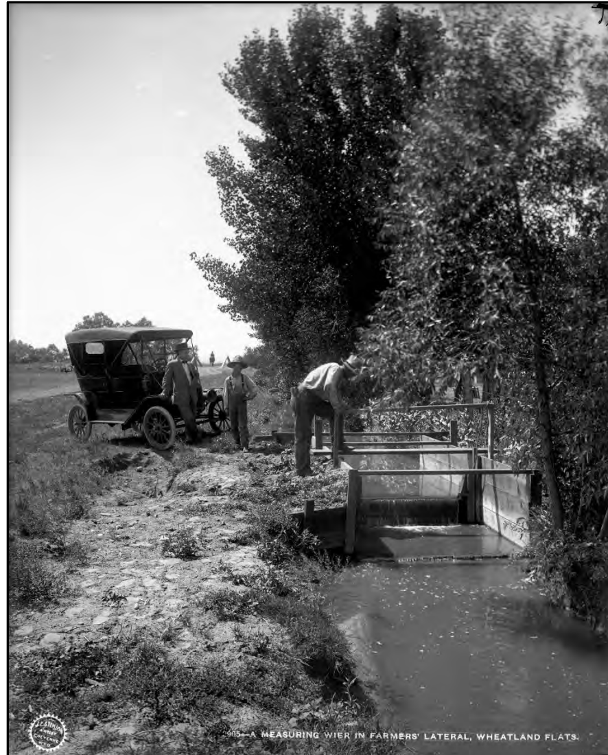
Figure 63. Historical photograph, circa 1909, of a weir along the Farmers Lateral near Wheatland, Wyoming. A measuring wier in Farmers' Lateral, J.E. Stimson Collection, STIMSON NEG 2905, Wyoming State Archives.
