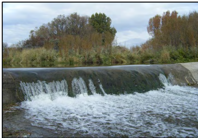
Figure 61. Example of a check drop on the Long Ditch in Converse County.
