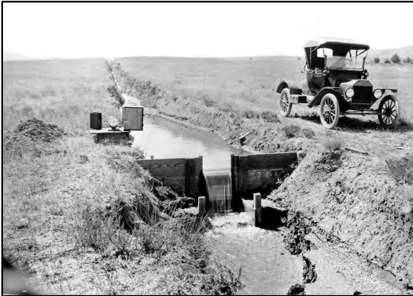
Figure 65. Example of a wooden drop structure, circa 1920s. Irrigation dam, Dams, SUB NEG 18828, Wyoming State Archives.
