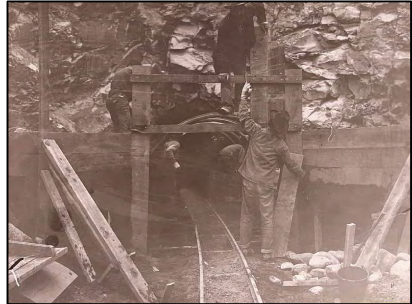
Figure 56. Construction of a tunnel on the Shell Canal, circa 1909. Image shows workers and forms used for the concrete tunnel structure. Tunnel portal Shell Canal, Canals Folder, C1226-48, Wyoming State Archives.
