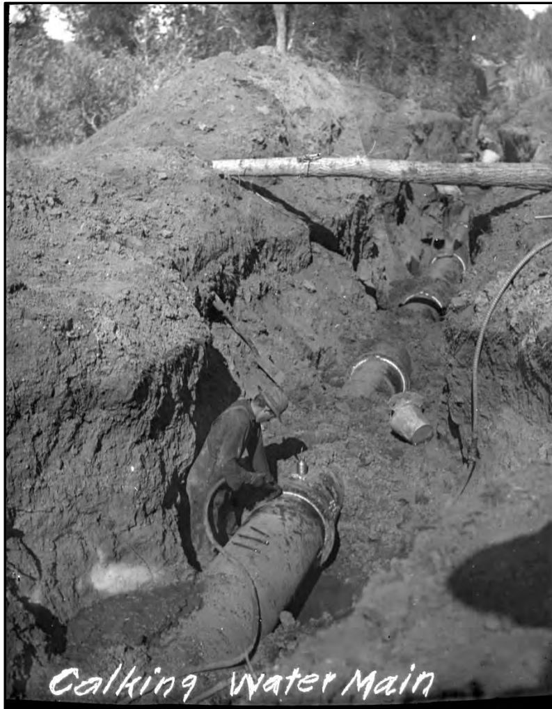
Figure 58. Historical photograph, circa 1910, of a buried water pipeline. Caulking water main, Lantern Slides, H55-53/074, Wyoming State Archives.
