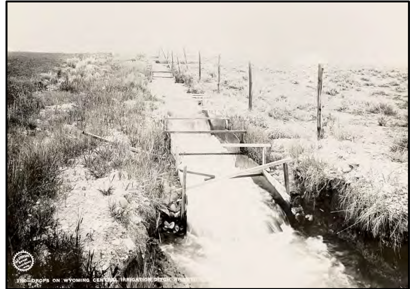
Figure 66. Series of drop structures on the Wyoming Central Irrigation Company's ditch, circa 1910. Drop structure Wyoming Central Irrigation Company, J.E. Stimson Collection, STIMSON NEG 3100, Wyoming State Archives.
