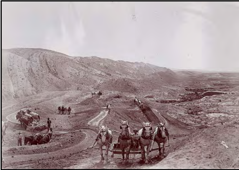
Figure 8. A 1908 photograph of grading work occurring during construction of the Shell Canal. Grading work on Shell Canal, Canal Folder, C1226-51, Wyoming State Archives.
