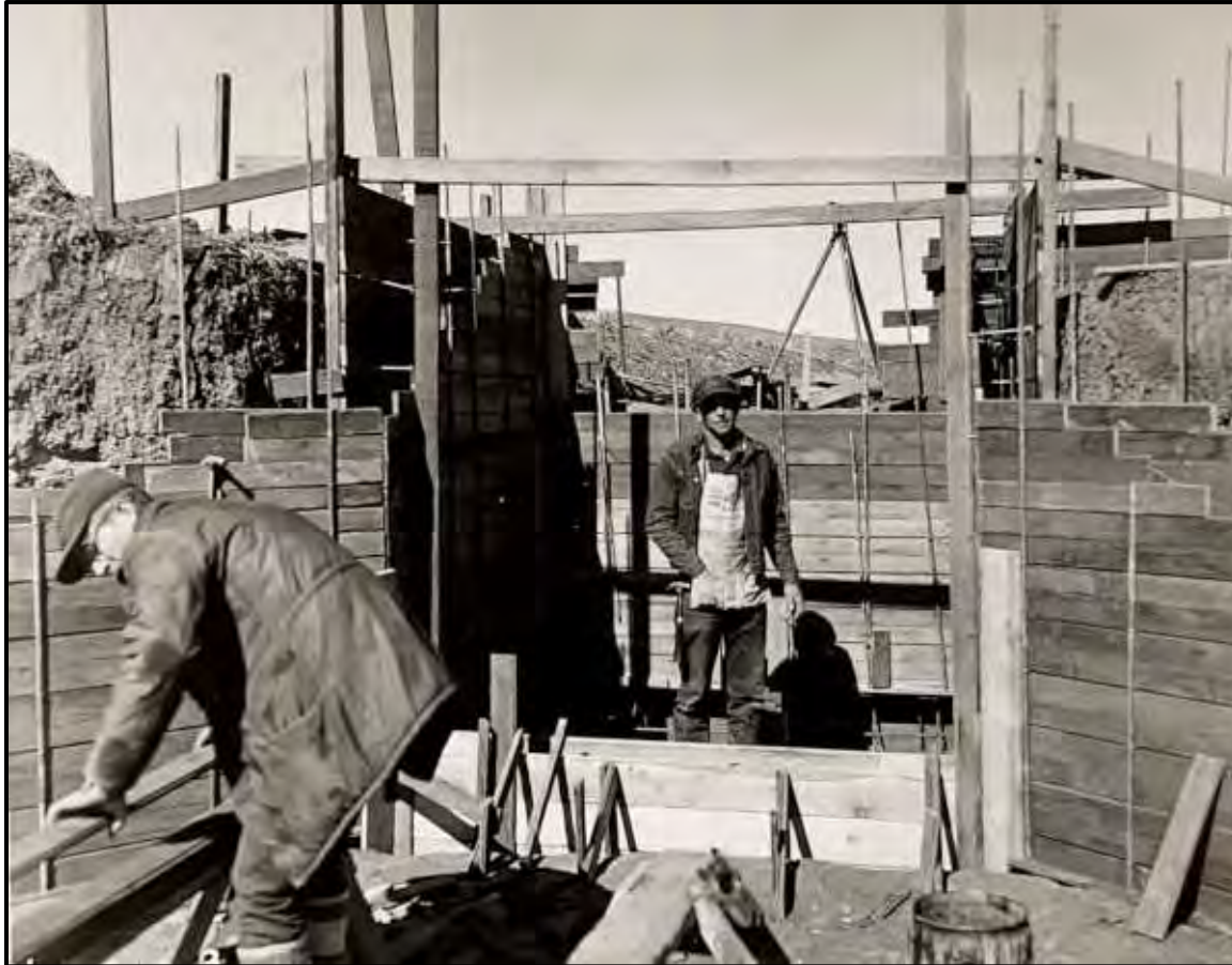
Figure 30. Workers constructing the wooden board-forms for the steel and concrete drop structure on the Cottonwood Canal, circa 1961. Drop structure construction, Department of Agriculture Collection, WY-6926-3, Wyoming State Archives.
