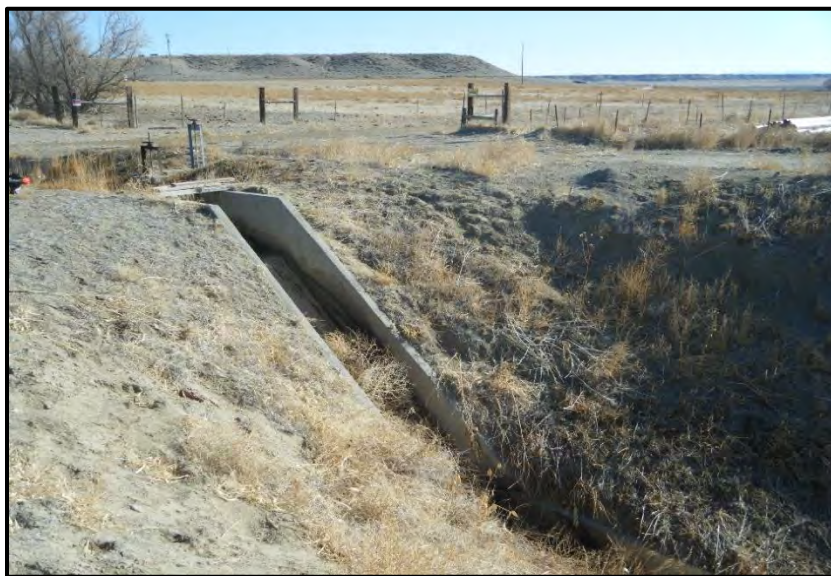
Figure 59. Example of a concrete drop structure, showing modern condition, on the Wyoming Canal Lateral 27.3 in Fremont County.
