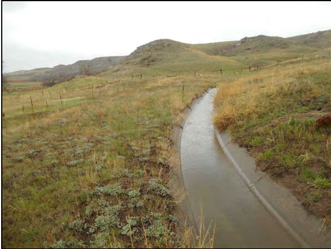
Figure 45. Example of a concrete lined ditch of the E 7 Ditch No. 1 in Laramie County.
