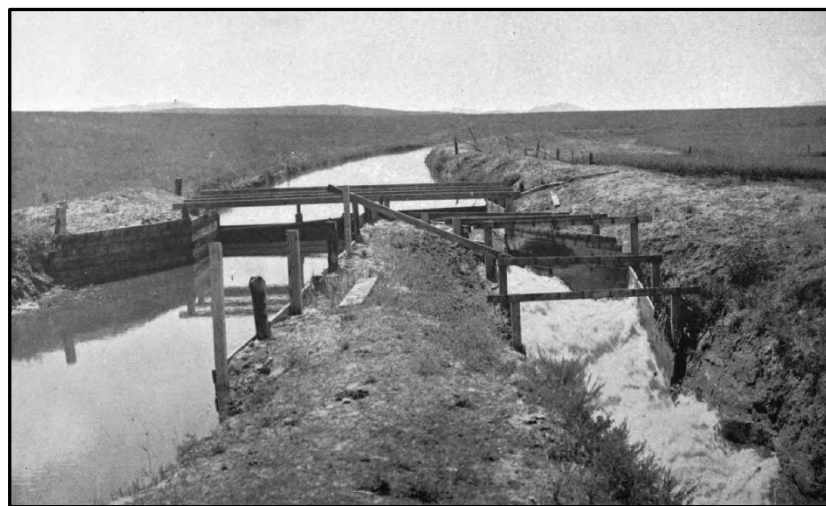
Figure 24. Historical photograph, circa 1908, of the Wheatland Industrial Company's Lateral No. 1 (right) diversion from Canal No. 1 (left) (Johnston 1908:42).
