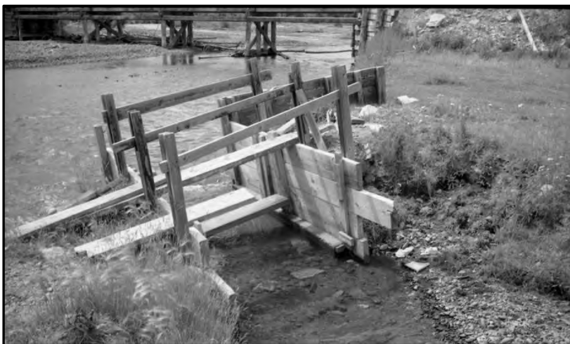
Figure 49. Undated historical photograph of a simple wooden outlet structure. Irrigation ditch gate, Wyoming Game & Fish Department Collection, P98-31/2051, Wyoming State Archives.
