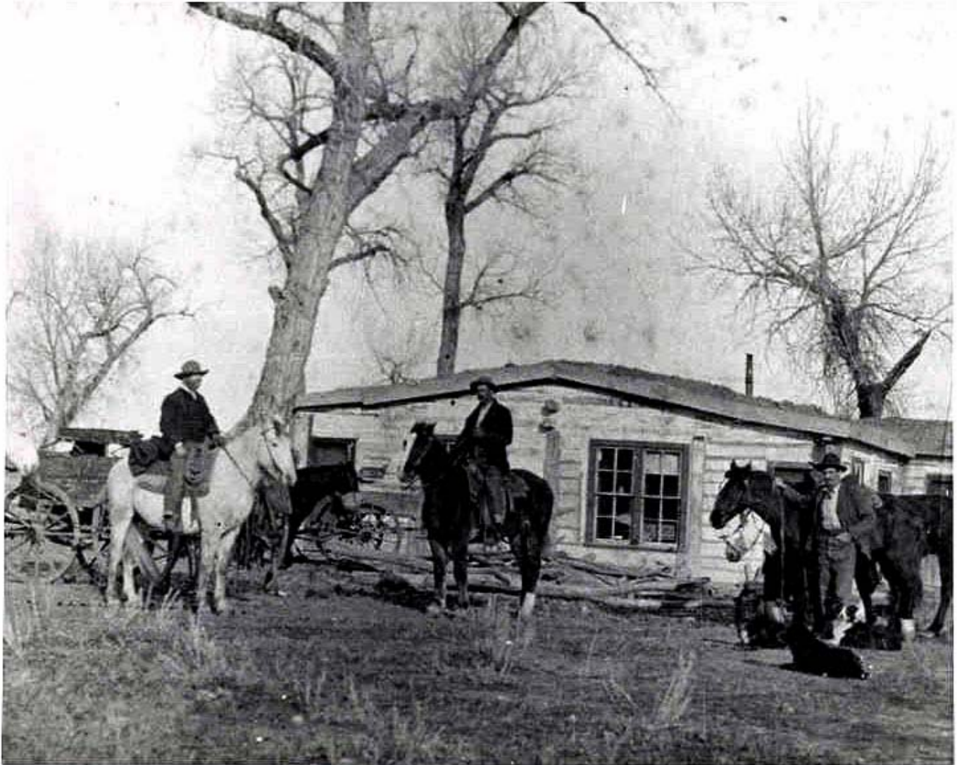
Scotch Outfit, Johnson County, 1909. The Scotch Outfit was one of the largest sheep operations in Johnson County. Photo: Johnson County Library Local History Collections. Note hewed logs, piece-sur-piece construction, and sod roof on the ranch building.
