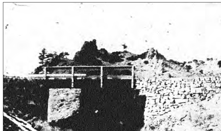
Completed CWA bridge on Hanna-Casper Road, showing rock-work and "unusually large clearance for floods." "Review of C.W.A.: State of Wyoming," Wyoming CWA Project Files, Reel 9, Document #22841.
