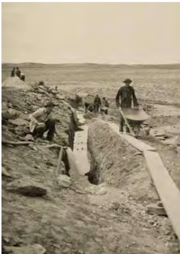
Building a puddle core for a dam.
