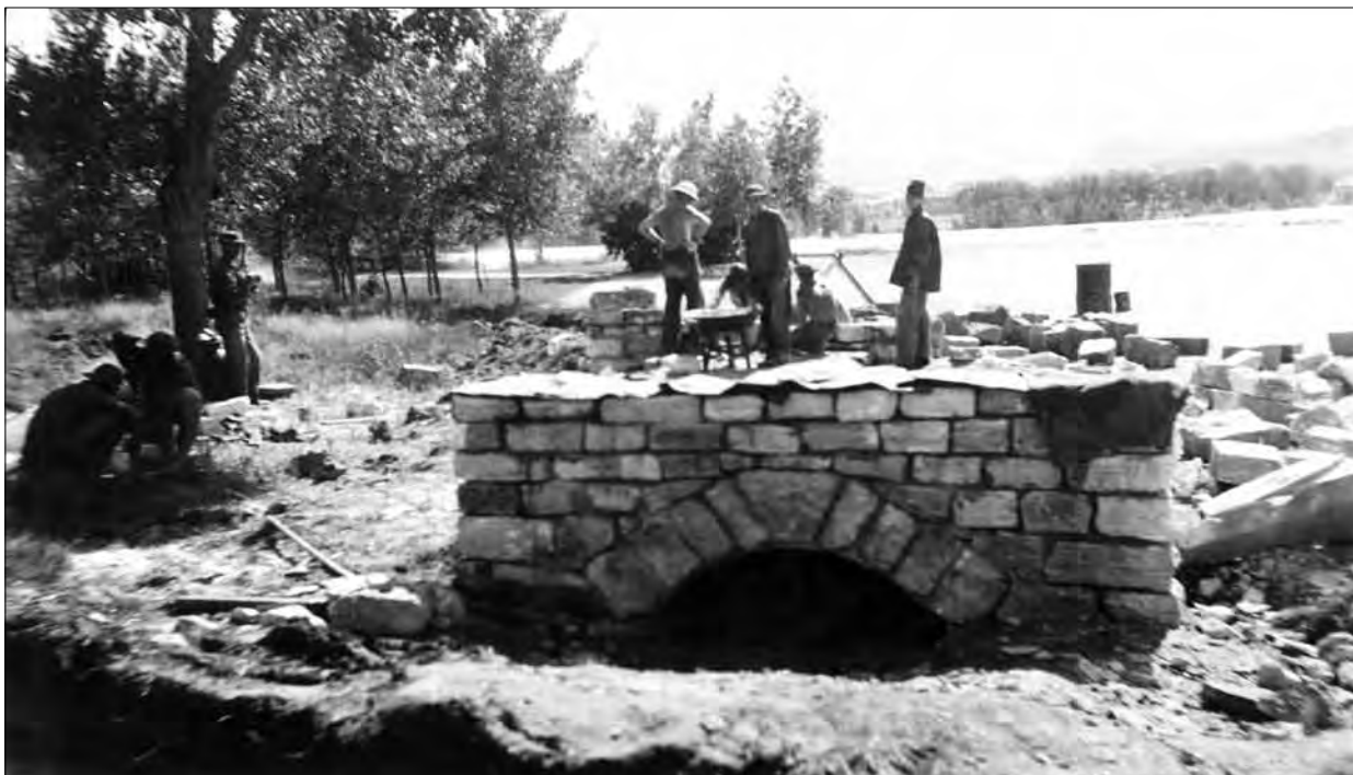
CCC workers building a stone culvert at Saratoga Hot Springs State Park. Courtesy the Wyoming State Archives, Wyoming C.C.C. Camps, 32B.
