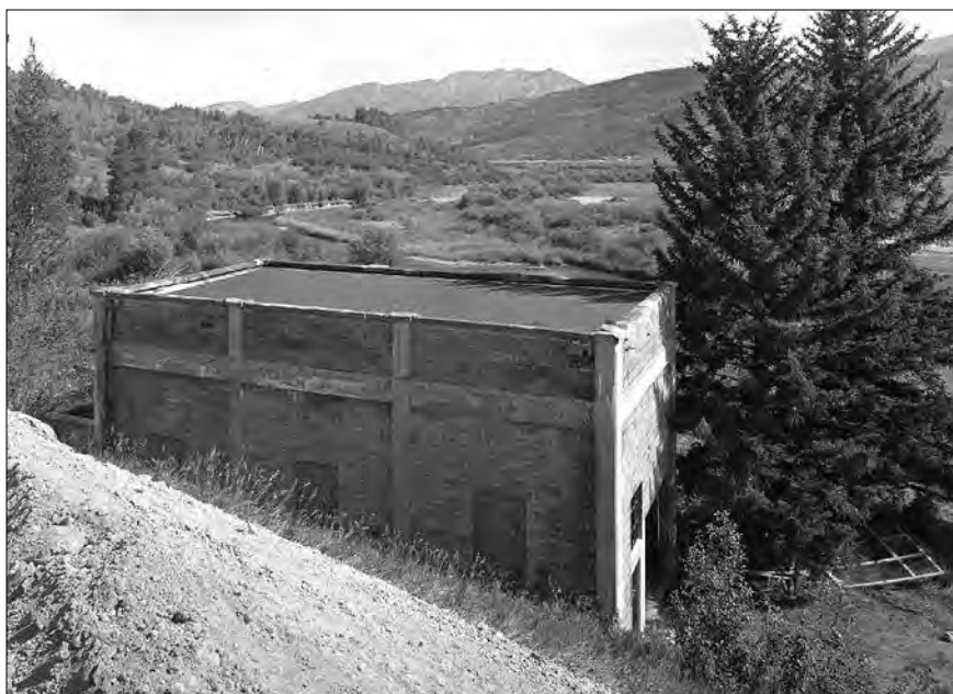
Salt River Hydroelectric Power Plant near Etna in Star Valley. Reportedly constructed with Rural Electric Association funds in 1938, this facility includes the building housing the power plant, a concrete inlet structure, an overflow spillway, and a tailrace canal leading away from it. Photograph by Richard Collier, Wyoming State Historic Preservation Office.
